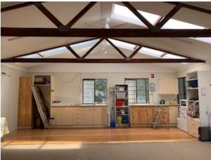
(New ceiling, insulation and skylights)
